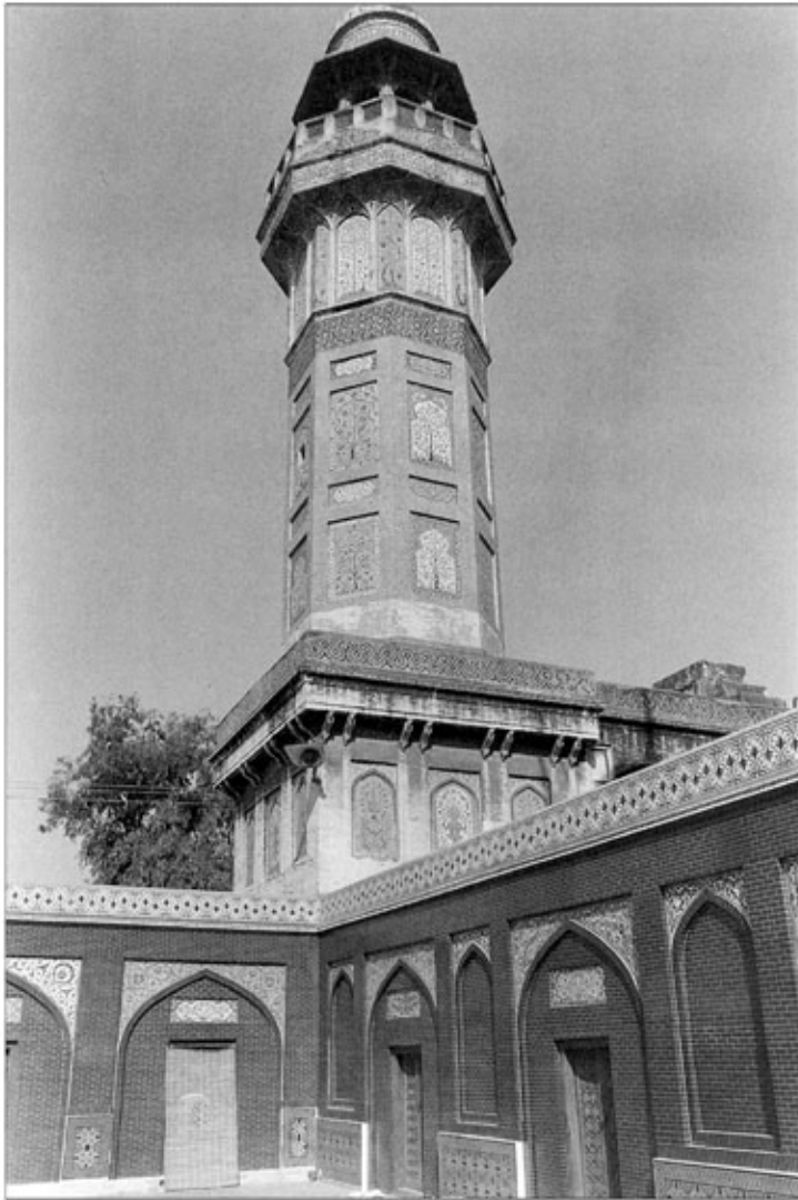
Minaret of the Wazir Khan Mosque, Lahore, Pakistan (above), and the minaret of the Yivli Mosque, Antalya, Turkey (right). The brick walls of the seventeenth-century Wazir Khan Mosque are covered with glazed-tile mosaic. The fluted fourteenth-century minaret of the Yivli Mosque is atypical of Turkish minarets, which generally are slender and pencil-shaped.
